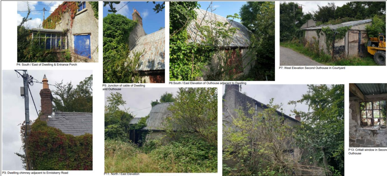
Figure 5.2: Extracts from MCORM Architects Dwg No. PL106 Demonstrating the Poor Condition of the Derelict Buildings on Site
