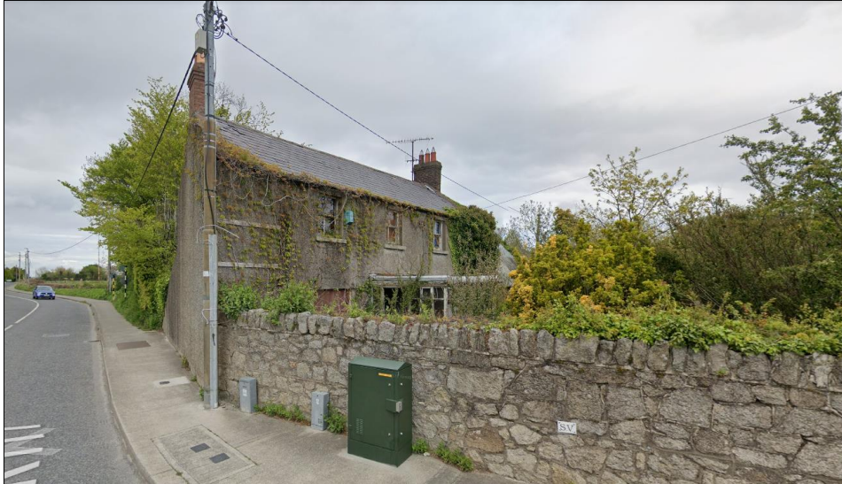
Figure 5.4: View of a Portion of the Derelict Buildings (Rockville dwelling) from Enniskerry Road with Dwelling Providing a Blank Gable onto Enniskerry Road
